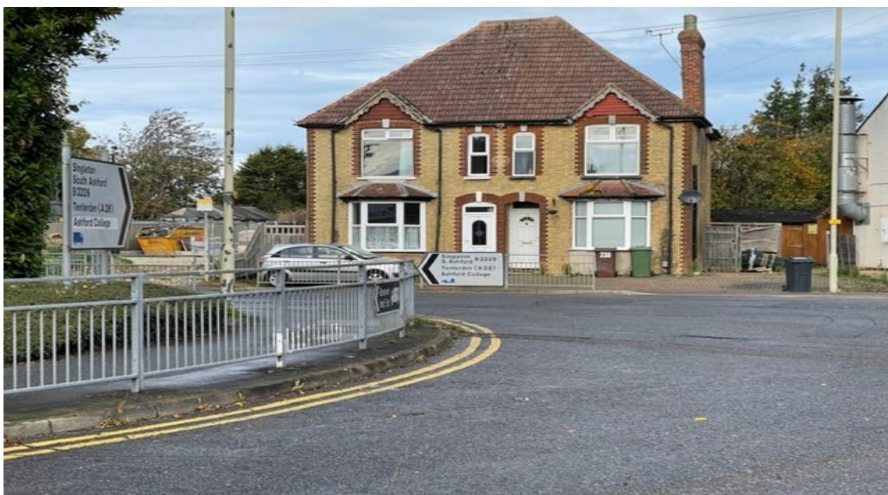
Figure 2: Photograph showing the pair of semi-detached dwellings
